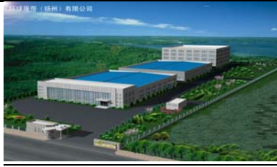
Global Track's Manufacturing Headquarters
